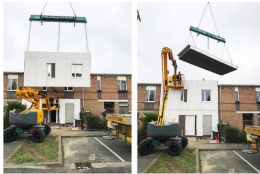
Source: BuidUp Offsite renovation
