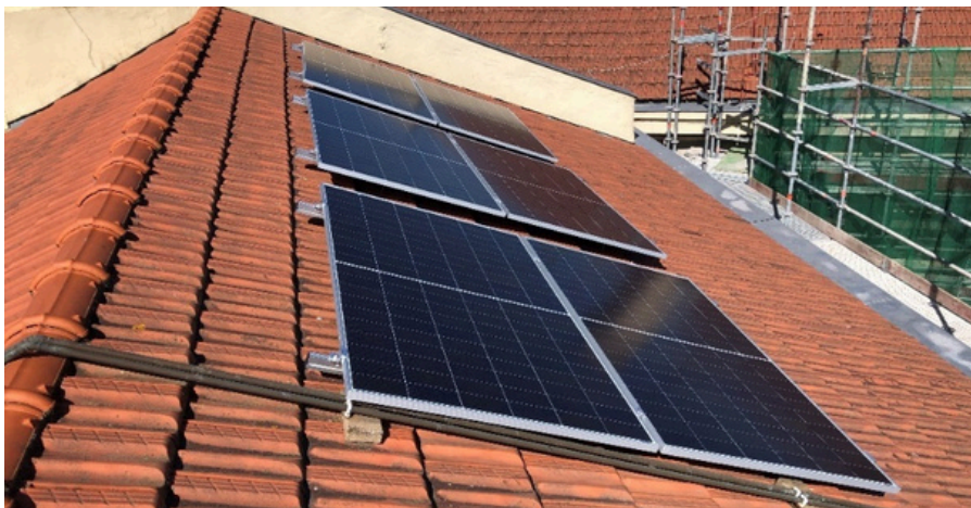
Solar photovoltaic panels installed on the roof of the TorreUrizar residential complex. Source: Bilbao Municipal Housing
