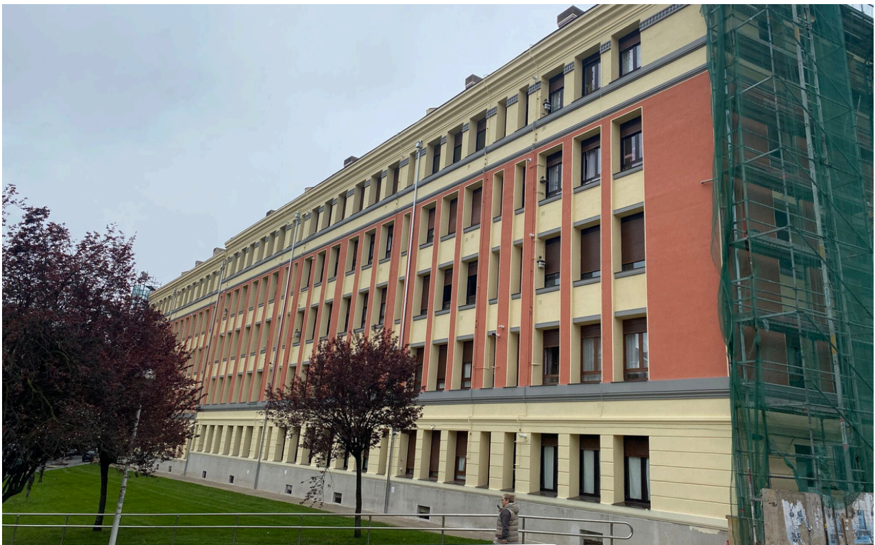
Outdoor view of the TorreUrizar building complex following the urban regeneration works. Source: Bilbao Municipal Housing
